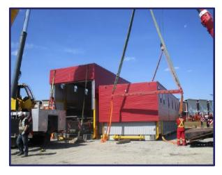
As noted already, a typical fire station has a life expectancy of 50 years before the cost/ benefit ratio starts to work against the municipality in terms of maintenance, basic function, and design. The EXTREME fire stations could meet that life cycle because they are made from steel and aluminum and additional modules can also be added if the station needs to expand its footprint.
